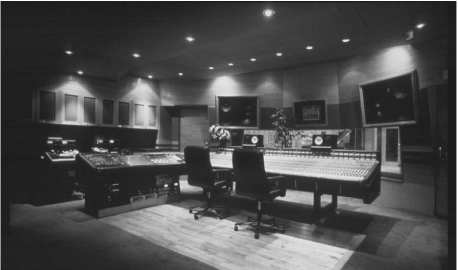
Figure 9.16. A Sam Toyashima control room at The Townhouse, London, having a hard front wall and highly absorbent rear wall.
